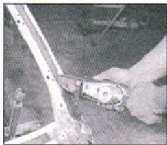
Removing paint and other coating in concave places.
